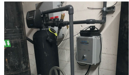
INSTALLATION: EasyWater Series C System — Model CLC-1000
