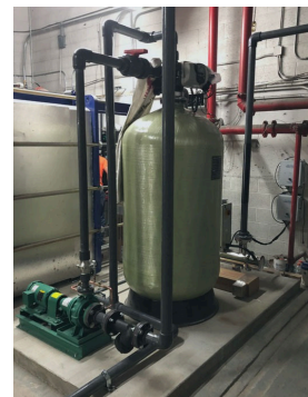
INSTALLATION: EasyWater CTF-100 Treatment System
