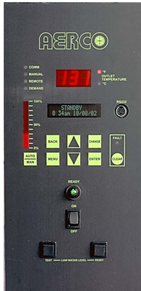
C-More Controller Front Panel
