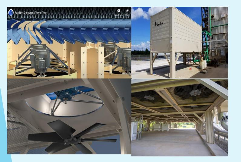
Bottom Fans-Safety, Longevity **Direct Drive** Motors-Maintenance, Safety Fan Array-Redundancy, Reliability, Flexibility, N+1 No Cranes Grade Level Simple Slab No Basin **NO Louvers**
