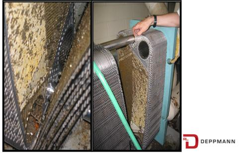
In a plate heat exchanger, the plates are very thin, and the passageways are small. The small passageways allow higher velocities. The higher velocities provide a better "U" value and more BTUH per square foot of heat transfer surface. This is a good thing.
