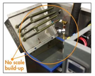
DriSteem Vapormist<sup>®</sup> humidifier heaters and tank after 200 days of non-stop runtime at 100% demand
