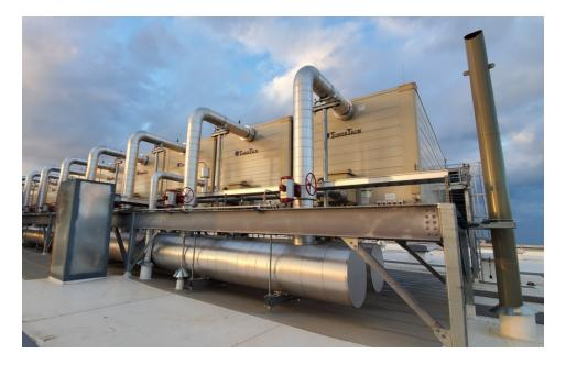
Tower Tech also contributes to saving lives. The unique low water storage volume reduced stagnant areas, and elimination of the large tower pan <u>reduces the growth of harmful</u> <u>bacteria</u>. The low drift also reduces the spray around the towers.
