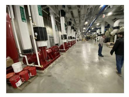
There were many applications using Bell & Gossett products. The cooling system uses Bell & Gossett vertical split case pumps. Since the plant is mounted on mother earth, there are no vibration eliminator pads under these pumps.
