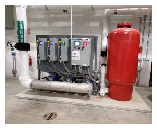
The cogeneration plant requires water. The proper water pressure can be critical to a variety of areas in the plant. The Ford Motor research and engineering campus has a wildly varying plumbing load. The range from low flow to full demand has a large effect on the water pressure. The CEP also has a varying load. The <u>Bell & Gossett Technologic pressure</u> <u>booster</u> is up to the task of providing constant water pressure with varying suction pressure and varying building loads.
