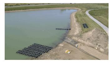
The water source heat pumps we normally see in the northern climates will use a geothermal system with the piping heat exchangers installed in pond/lake water or in an in-ground earth coupled system. <u>The</u> <u>photo above is from Contractor Magazine</u> and features a water source system
