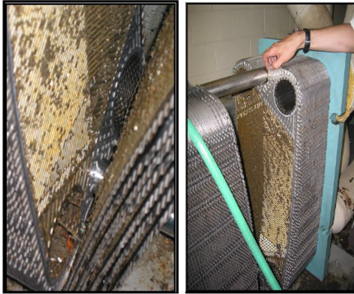
Fouled plate heat exchanger. Photo provided by James M. Pleasants Company.
