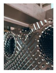
Four holes punched in the plate corners form a continuous tunnel which acts as a distribution manifold for the inlet and outlet of each fluid. Each plate is fitted with a gasket. The gasket either confines the fluid to the port or directs the fluid to the heat transfer area of the plate. In a single wall design, the two fluids are separated by these gaskets.
