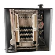
Each of the tubes shown above can be individually replaced. This reduces the material cost. The labor to replace the tubes does not require a lot of technical training. It can be done on the jobsite with minimal lead time and service time. Bryan has an older manual, <u>Instruction</u> <u>34</u>, that has the steps.
