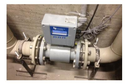
Traditional hydronic and plumbing flow meters with BMS capability have restrictions on the location in the piping system as well as the types of fittings and valves in front of them. The very forgiving inline mag meter has traditionally required enough pipe diameters to be a challenge at times. This is the required amount of straight pipe before and after the device to ensure accuracy.
