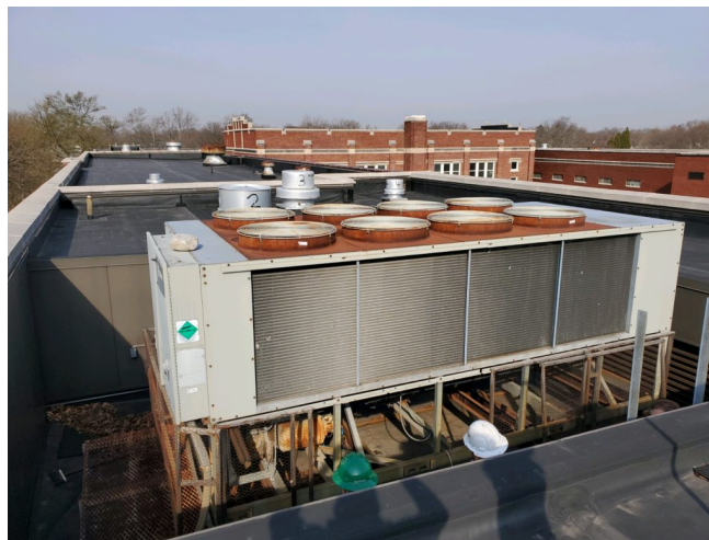
BirminghamPierce Middle School Chiller
