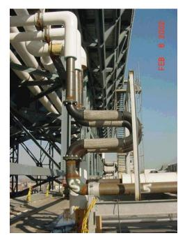
Possibly a pump is not on a variable speed drive or soft starter. When the pump starts up there may be a thrust load pushing up. The thrust anchor on the header should be designed to handle this, but what if they put spring hangers up there? Something is going to try to move.
