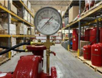
The standard Bobco Gauge Package is designed to give the most accurate gauge reading possible on a centrifugal pump. Differential pressure gauges can greatly reduce system operating errors, improve system efficiency, protect expensive equipment, and reduce maintenance time. The standard Bobco kit will come with a Miljoco 4.5" stainless steel contractor gauge with a 30, 60, or 100 PSI gauge.
