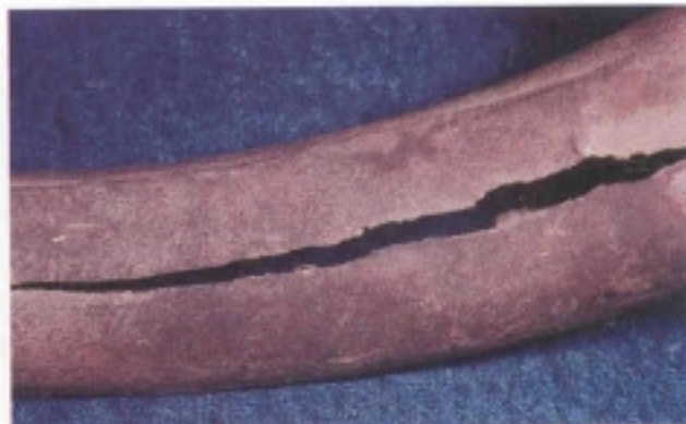
Fig. 10. Thinning of tube because of general corrosion.
